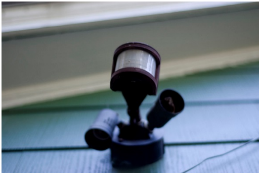
Property owners can connect their outdoor lights to motion detectors. These low-cost devices can help discourage crime by making it harder for lawbreakers to hide. Photo source: Joey Parsons.
