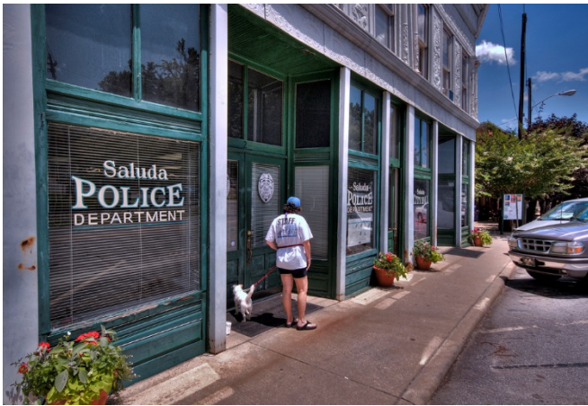
By establishing small neighborhood stations, especially in an existing vacant space, a law enforcement agency can improve its accessibility and be more visible to the community. Photo source: Frank DiBona.
