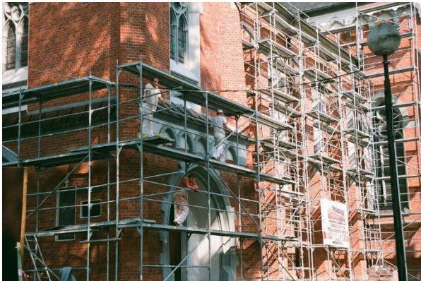
Facade renovation project. Photo source: PublicDomainPictures
