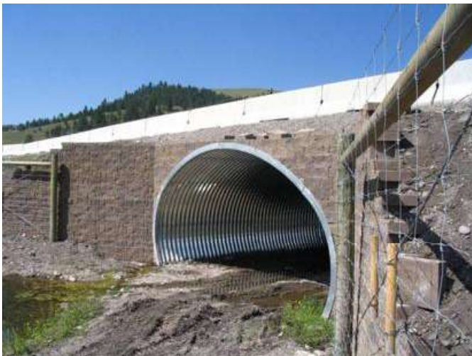
Example of a wildlife corridor underpass under a major road. Photo source: FHWA.
